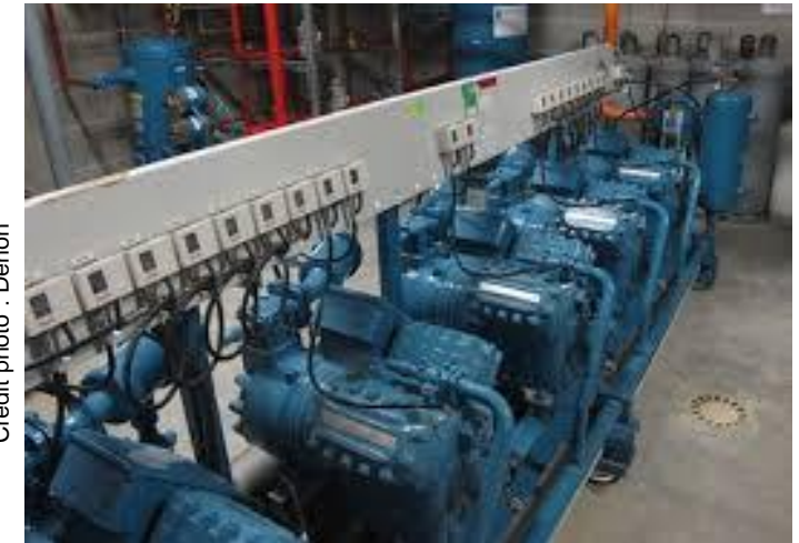
Typical rack of compressors working with low GWP blend
