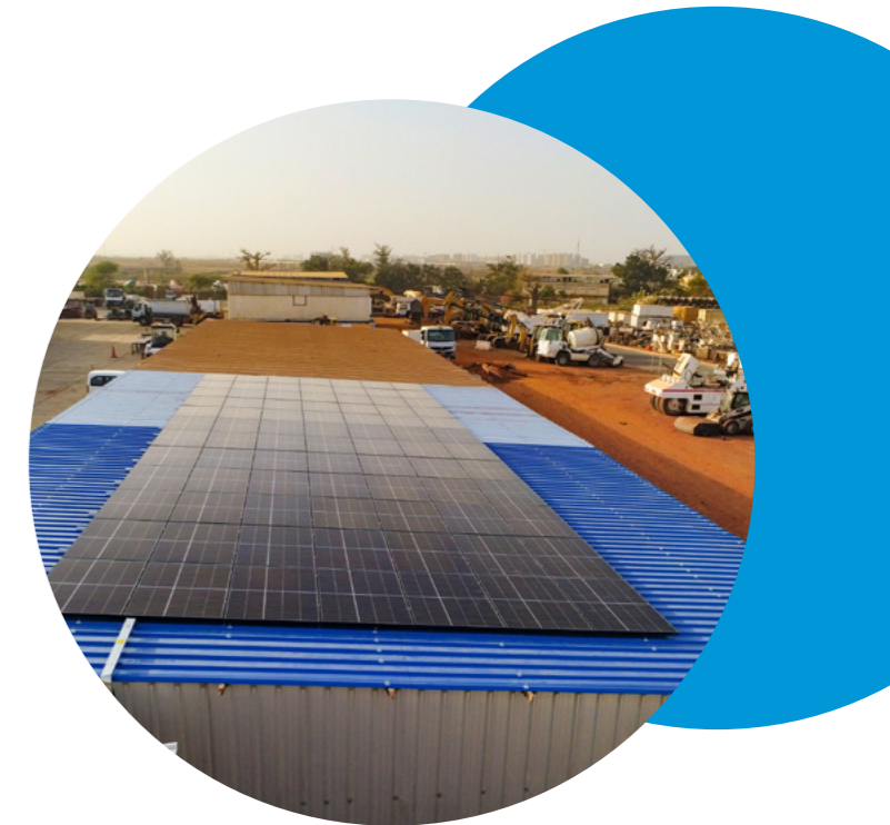
Solar panels installed at Eiffage Sénégal
