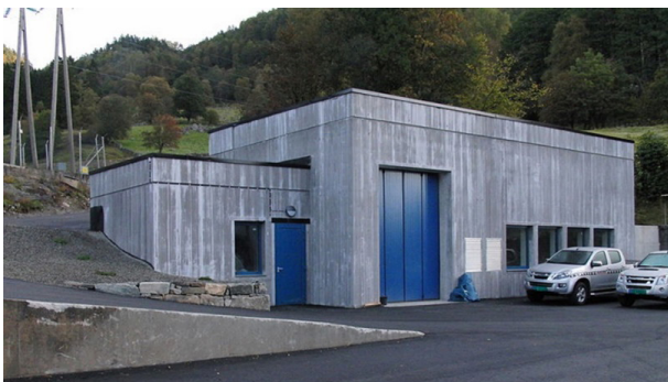
Figure 2. Haukland Power Plant
