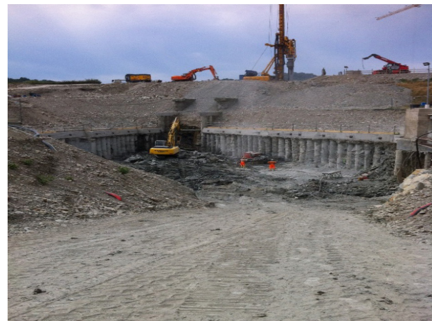
Figure 4. Working phases: (a) building of secant poles
