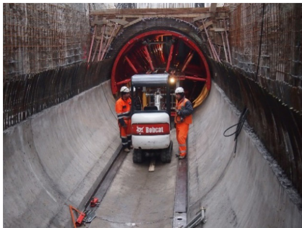
(g) second phase of concrete casting
