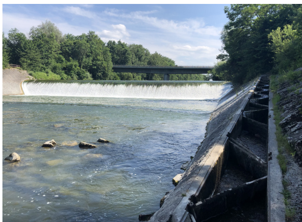
Figure 4. The Iller-weir Dietenheim before and after the Construction of the HSPP
