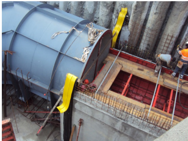
(g) second phase of concrete casting
