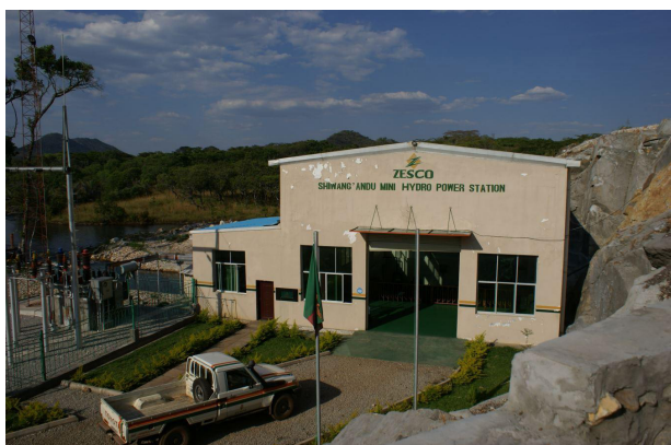
Figure 3. Shiwag’andu SHP plant
