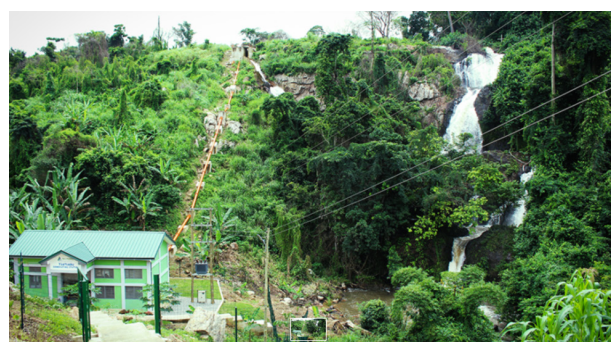
Figure 2. First small hydropower plant in Ghana
