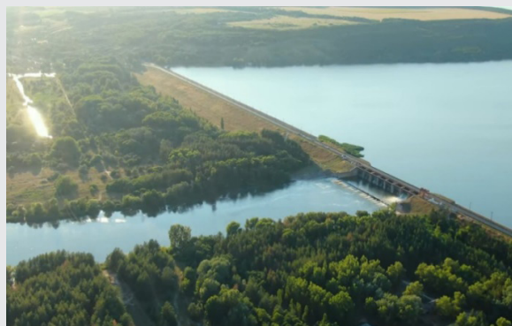
Figure 2. Hydraulic structures of the Pecheneg Reservoir on the Siverskyi Donets River, Kharkiv region
