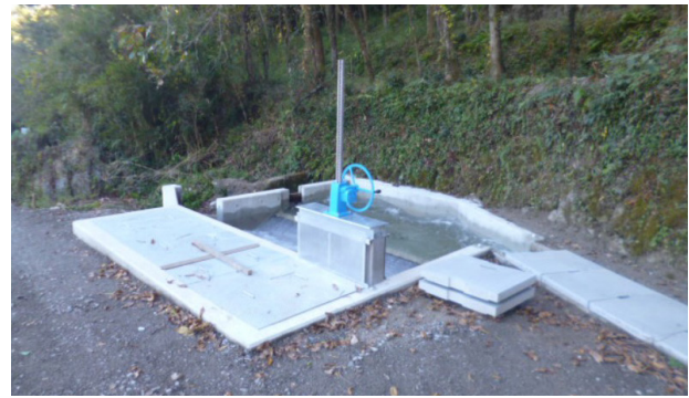
Figure 5. Newly made forebay tank on the existing water channel
