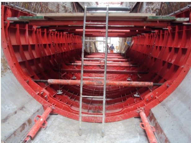
(e) first phase of concrete casting
