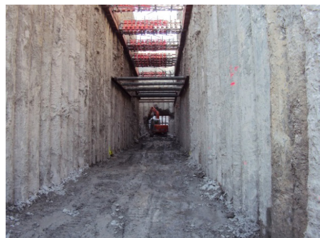
(b) support and excavation
