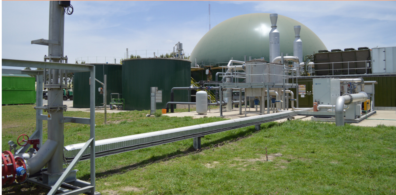
Biogas plant in Naivasha, Kenya. (Source: Vegpro)
