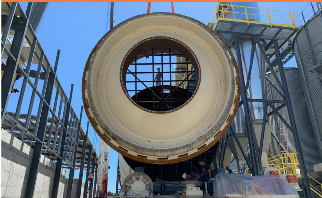
Installation of drying/torrefaction unit. (Source: Futerra Fuels)
